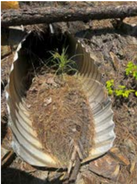
Outlet laden with pine needles
