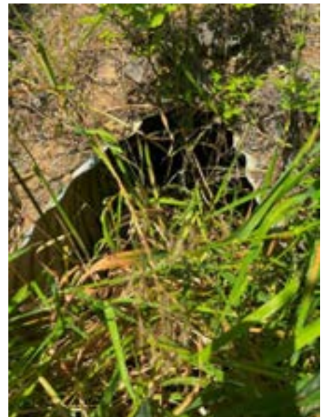
Outlet covered with dirt and plants
