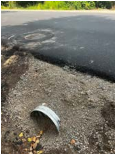
New culvert downstream of old outfall 1
