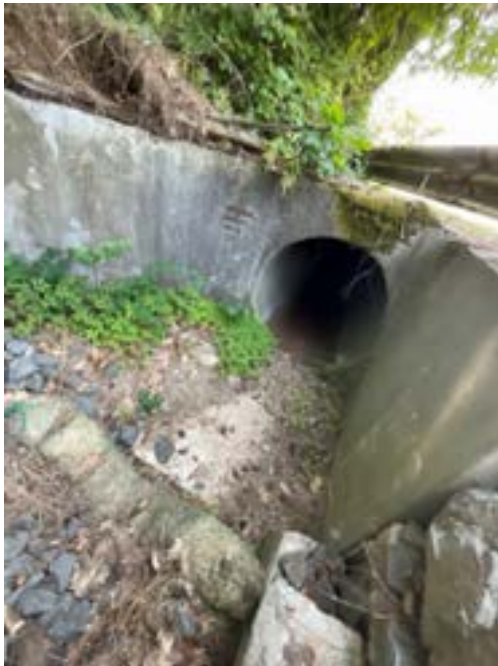
Open channel leading to culvert
