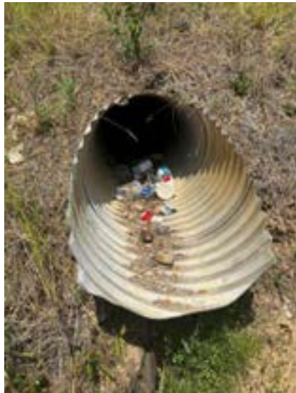
Litter scattered in culvert
